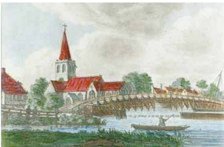
Old wooden bridge at Marlow with eel buckets attached, early 1800s
